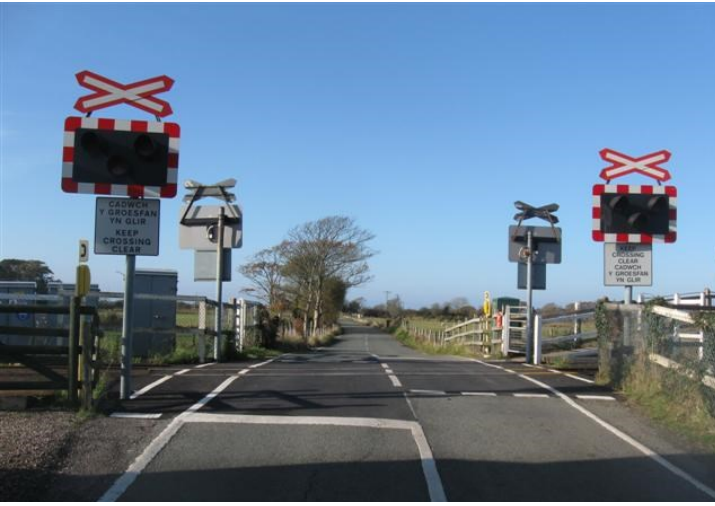
Talwrn Bach level crossing
