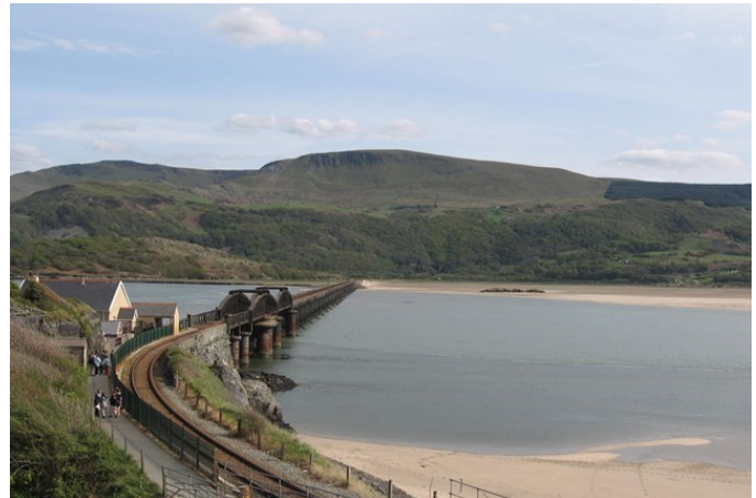
The iconic Barmouth viaduct was temporarily closed to rail passengers after a fire last month
